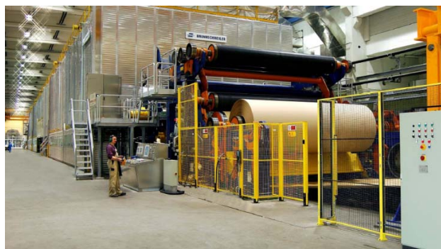
Figure 15. Paper plant in Spremberg [10]
